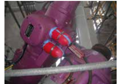
Alloy 825 MI wiring cable with KMASS gland protector can survive in the flash fire
