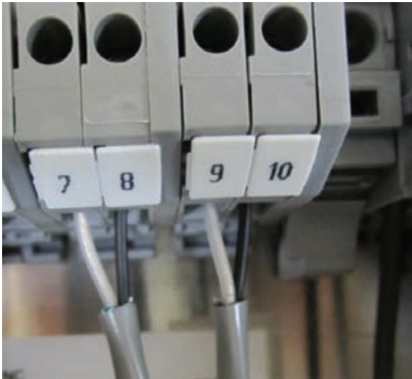
Two wire RS485 connection to host system at terminal blocks 9 (+) and 10 (-) in the TT-TS12-PANEL-xx versions
