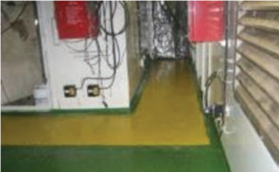
Figure 12. Heated Walkway
