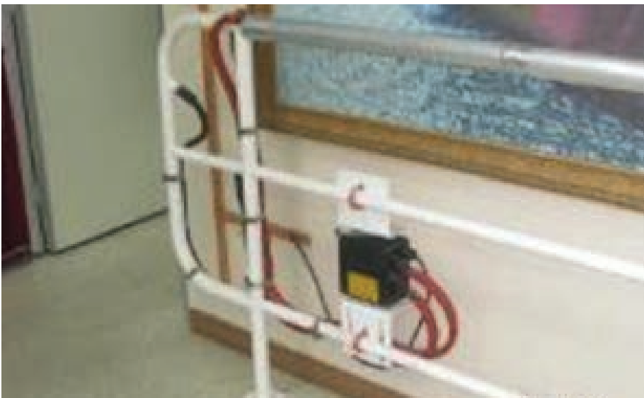
Figure 13. Heated Handrails
