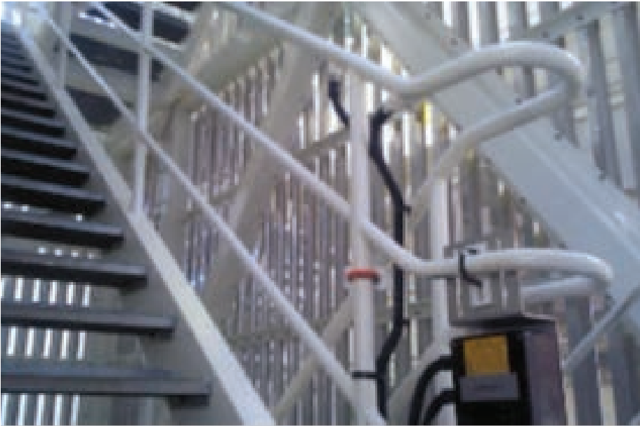
Figure 14. Heated Handrails
