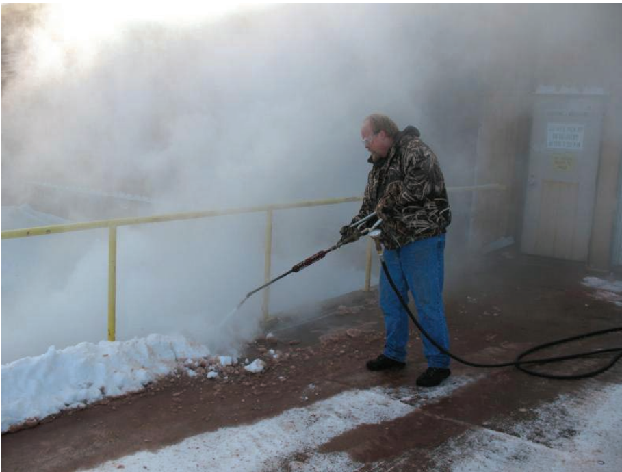
Figure 9. Ice removal using steam wands.
