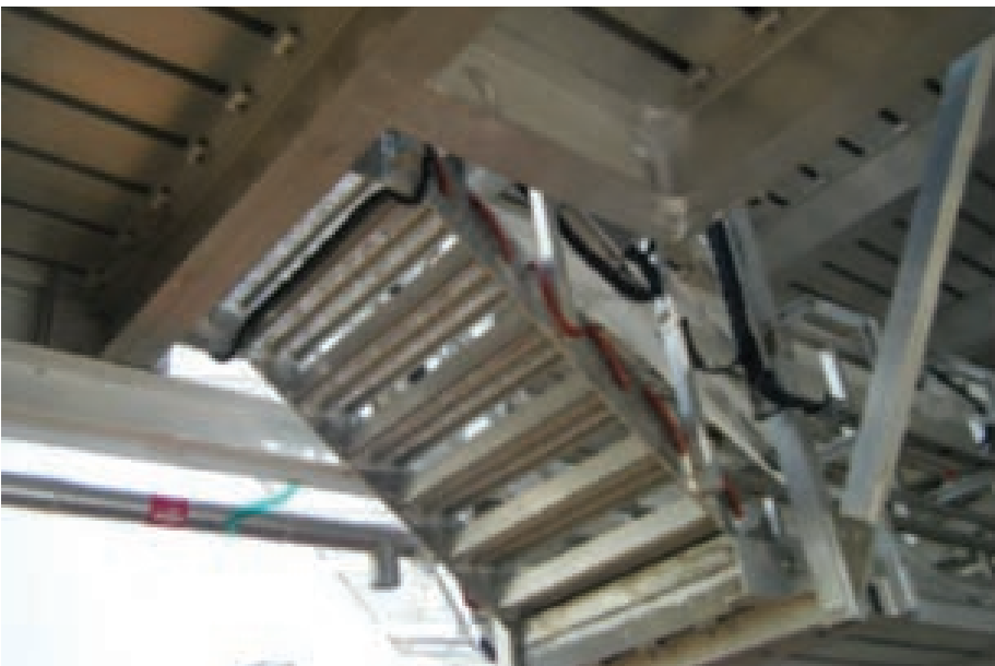
Figure 15. Heated Stairs
